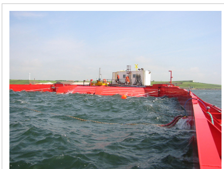
Wave Dragon seen from reflector, prototype 1:4½
