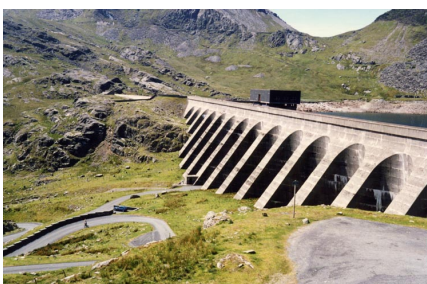
The upper reservoir (Llyn Stwlan) and dam of the Ffestiniog Pumped Storage Scheme in north Wales. The lower power station has four water turbines which generate 360 MW of electricity within 60 seconds of the need arising. The size of the dam can be judged from the road below.
