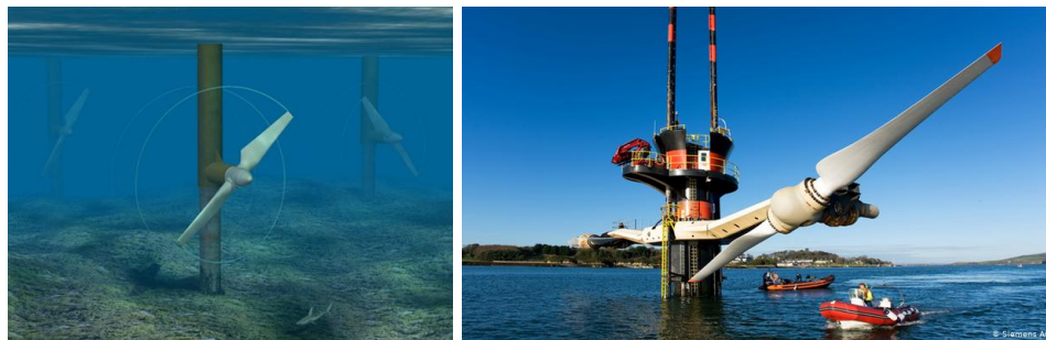
Figure 7.8: Tidal hydropower plants. Left: schematic draw of a tidal hydropower farm; right: a tidal power generator in Northern Ireland (1.2 MW).
