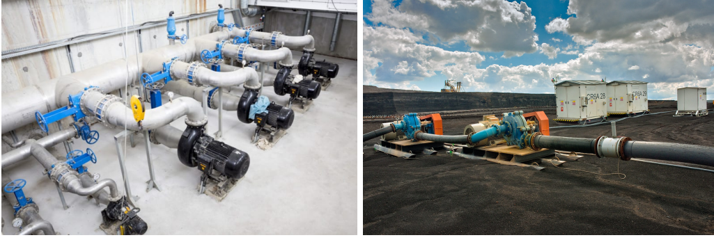
Figure 5.3: Pump stations with pumps connected in parallel (left) and in series (right).
